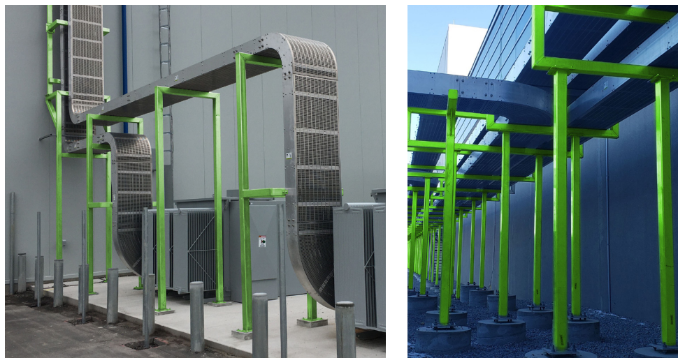
Disclaimer: Not actual colour. Green colour is used to highlight the supports
