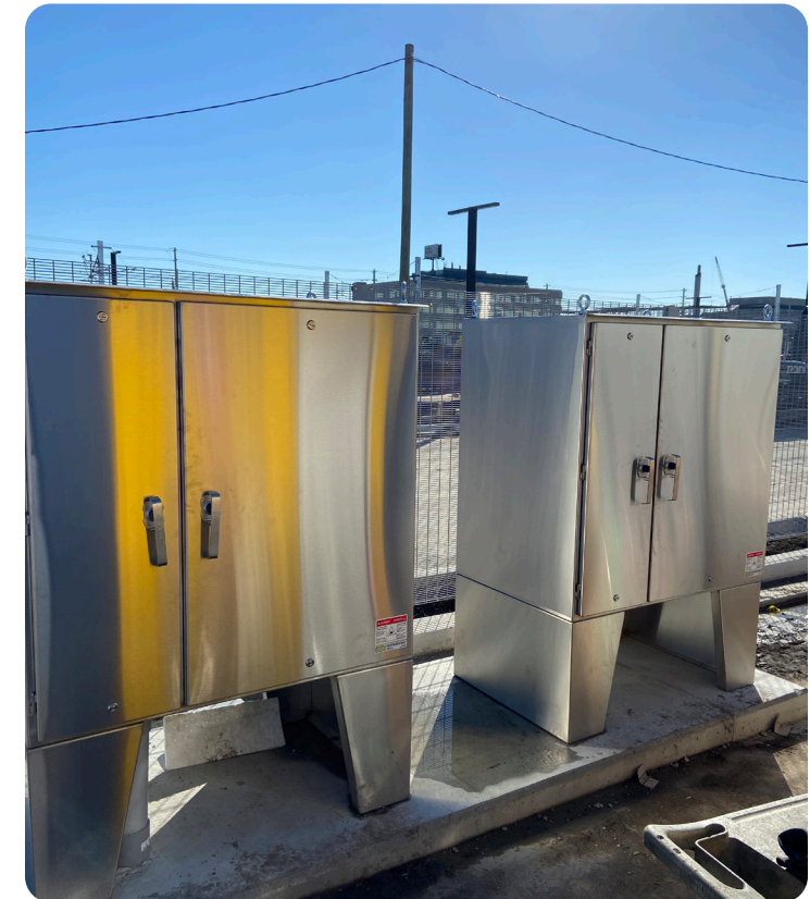
Double 600V 2000A Stainless Steel QC Panel
