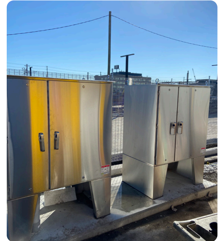
Double 600V 2000A Stainless Steel QC Panel
