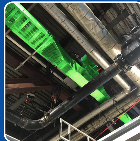
Installation - Custom Fitting Highlighted
