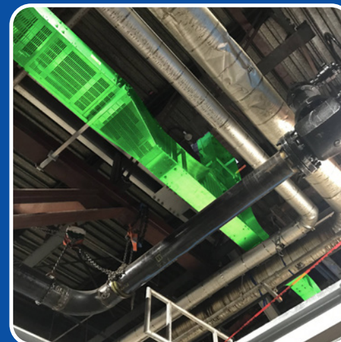
Installation - Custom Fitting Highlighted
