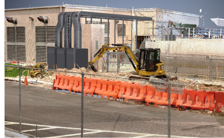
Power Bus Way cable bus model placed into 3D Scan point cloud
